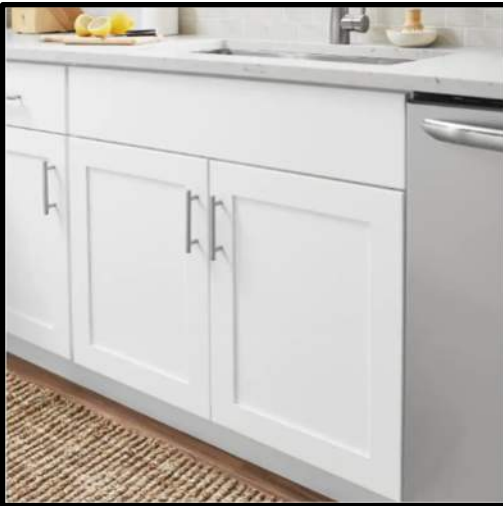
Kitchen Cabinets (base and walls)
